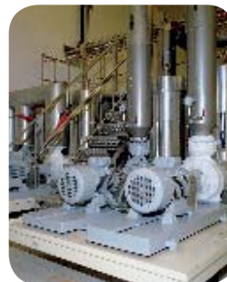
Pumps, compressors, fans
