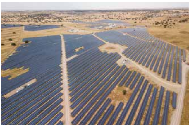
PORTUGAL Ourique, 46 MW HEC V1500 PORTUGAL'S 1 ST 1500V INVERTER
