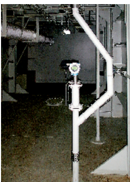
Microplit M FMR240 Misura in tubo sonda
