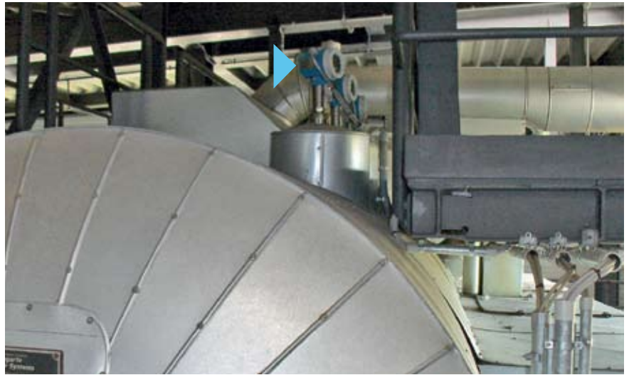
Level measurement in the steam drum with Levelflex M FMP45 (2 out of 3 installation) Level steam drum
