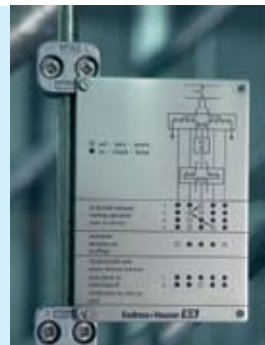
Operating instructions for 5-valve manifold
