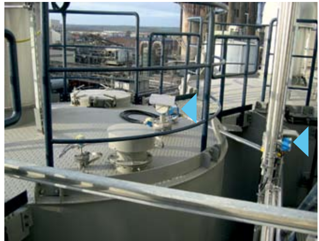
Level measurement of pulverized lignite coke using Levelflex M FMP40
