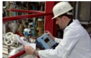
On-site calibration of pressure devices
