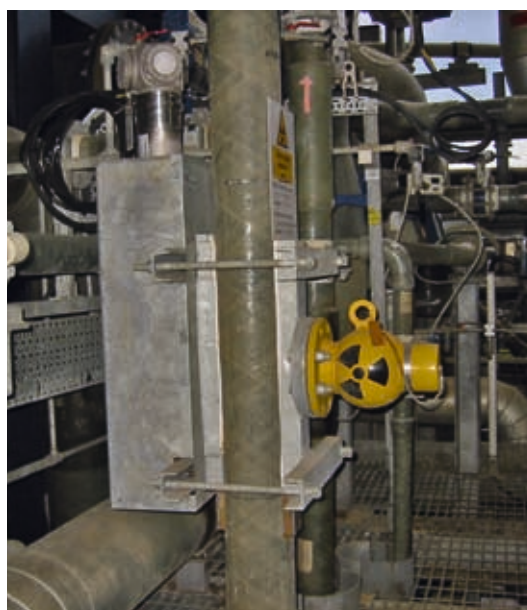
Gammapiilot installed in the main absorption cycle
