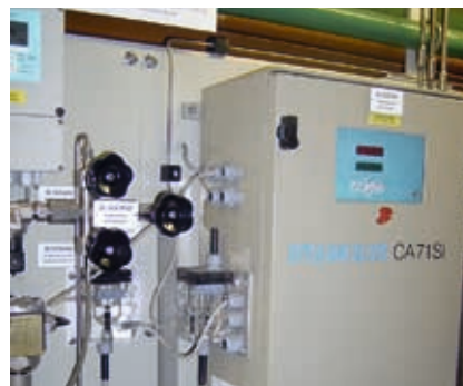
Stamolys for the control of silicate to protect the turbine
