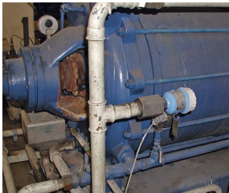
Liquiphant installed to protect the pump from running dry
