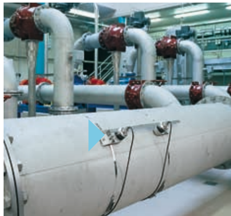
Prosonic Flow (clamp on version shown) is used to control cooling water for the main condenser
