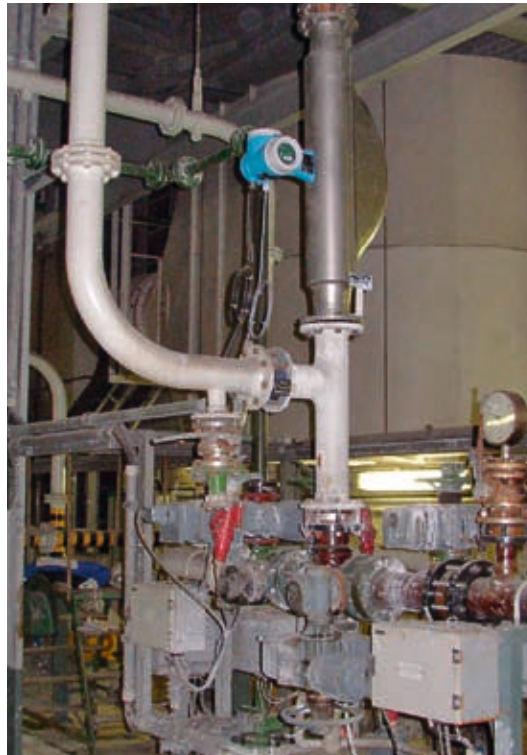
Promass installed in the main absorption cycle
