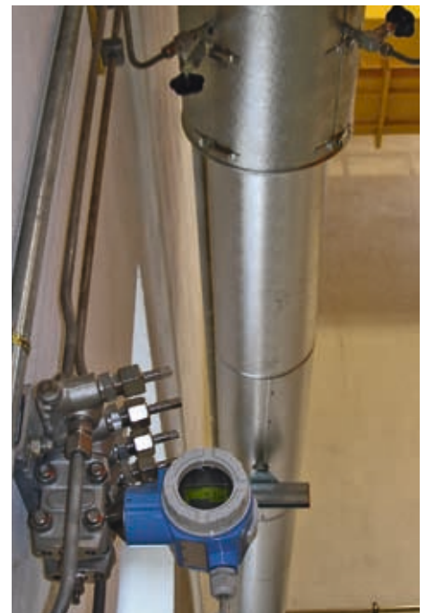
Deltatop (Deltabar S with primary element) for measuring superheated steam
