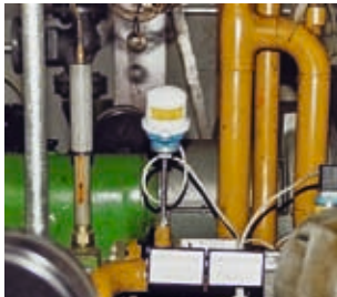
The Omnigrad resistance thermometer monitors the lubricating circuit at the cooling water pump
