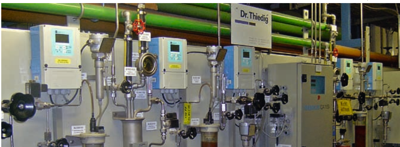
Sampling system with pH, conductivity and silicate
