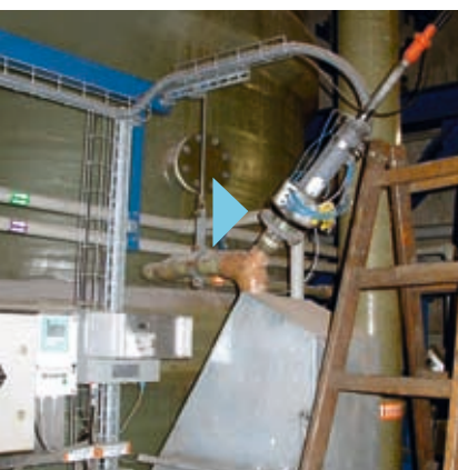
TopCal system in pH measurement for automatic cleaning and calibration
