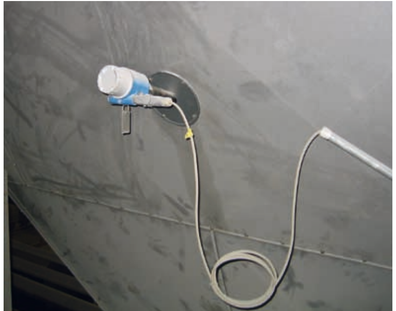
Capacitive sensor for maximum limit detection in the electrostatic filter
