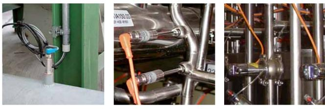
Monitoring of a supply pipework using compact thermometers and temperature switches
