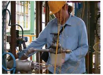
Maintenance of an installed diagnosis chamber
