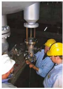
Installation of a multi-point thermocouple
