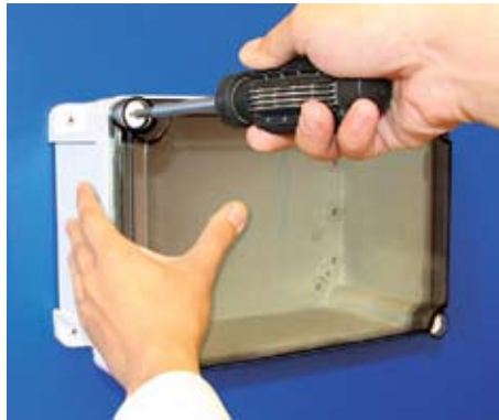
Fix the box on wall
