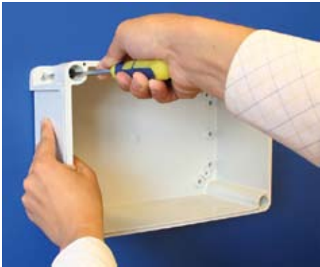
Fix the box on wall
