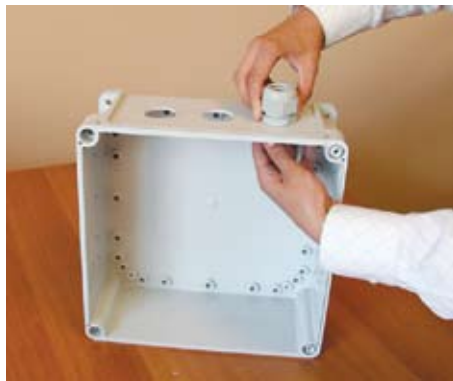
Install cable clips
